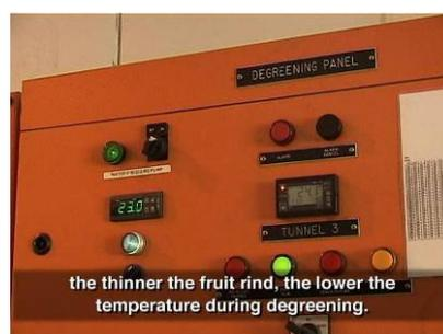
Temperature is very important and the rule is: the thinner the fruit rind, the lower the temperature during degreening, even though degreening is better at higher temperatures. Satsumas are degreened at 18-21°C; Clementines, Novas and Mandarins at 19-22°C; navels and other oranges at 21-24°C; grapefruit and lemons at 23-25°C.
