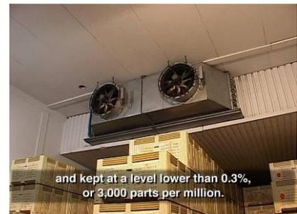
To protect fruit from high CO<sub>2</sub> levels, CO<sub>2</sub> must be extracted by ventilation fans regularly from the chamber, and kept at a level lower than 0.3%, or 3,000 parts per million.
